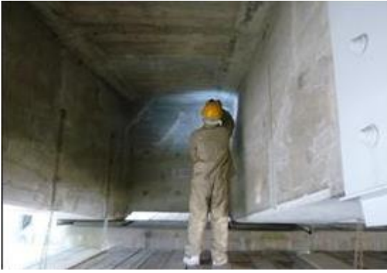
Figure 1. Photographing by a labor on a temporary scaffold deck for a visual inspection.
